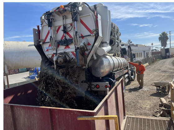
Hydrovac truck offloading — Gardena Recycling Facility
